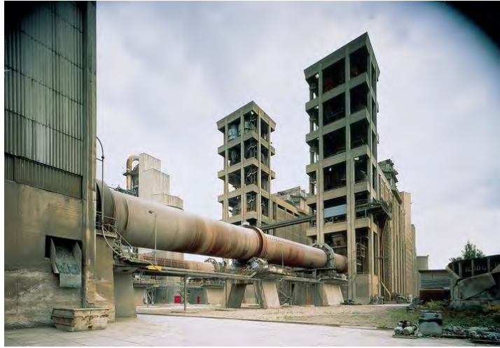
Figure 13.1: Two rotary cement kilns. We can see the cooking tubes —the kiln itself— and the preheating towers. The cooler can be slightly seen at the left.
